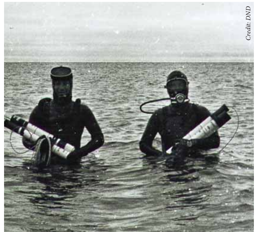
Divers about to lay Nitron charges to blast an obstruction at DEW Line site PIN-3 (Lady Franklyn Point, Victoria Island, Nunavut), July 1967.
